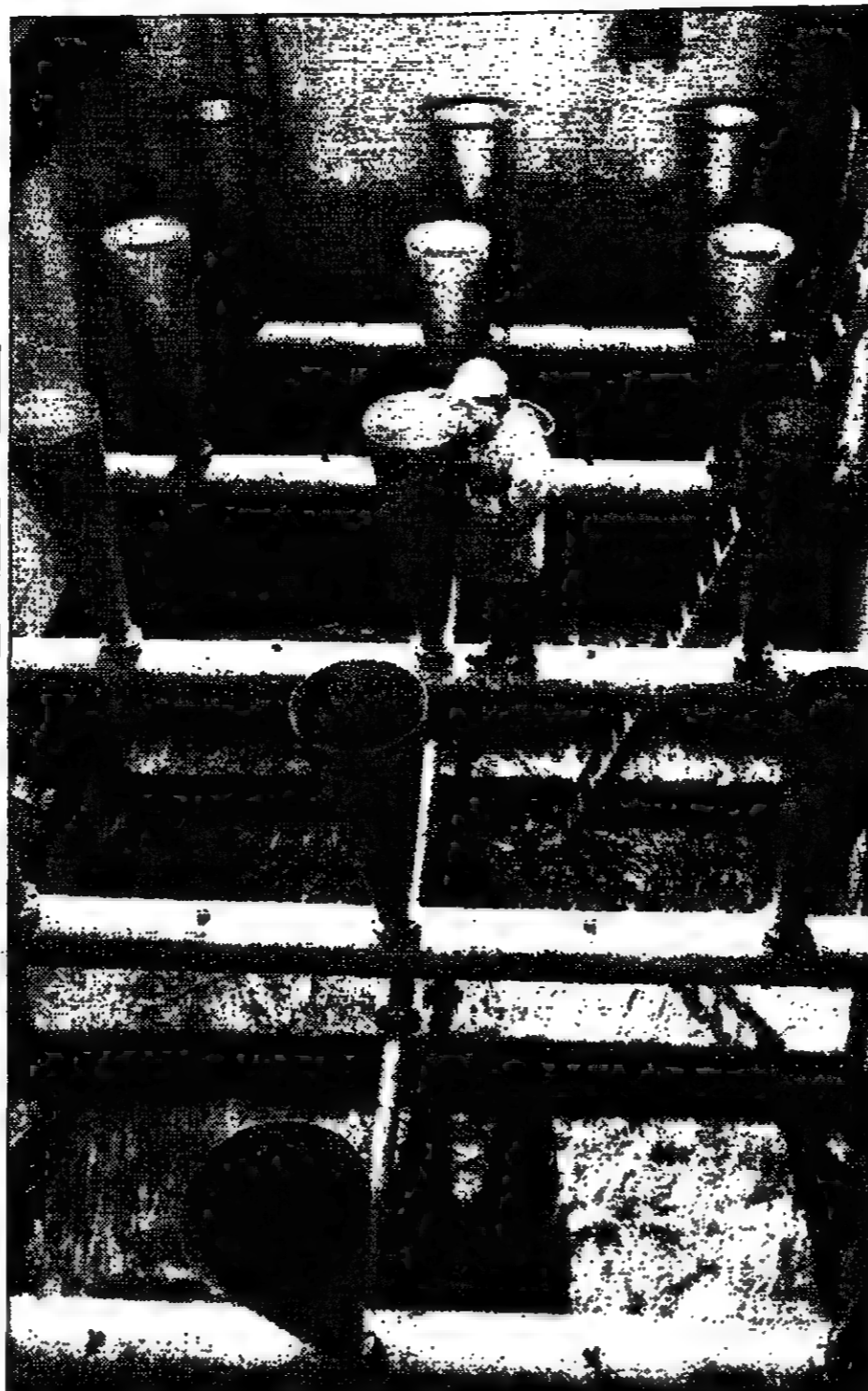
Suitable place for treatment... Thames' £40m new Walton plant PHOTOGRAPH BY DAVID HANSELL
